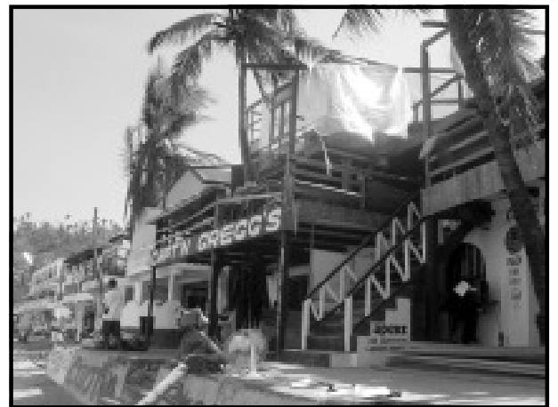
Capt'n Gregg's in Sabang lost a part of its roof
